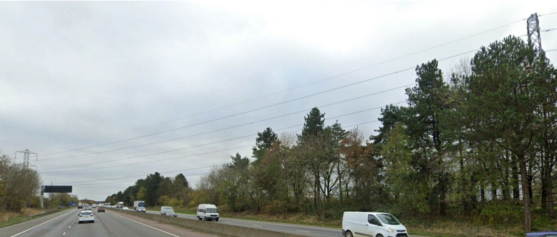
Figure D.1 – M1 motorway crossing at span ZL145-ZL146
