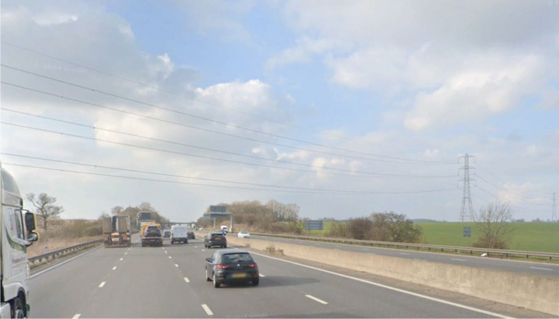
Figure D.2 – M1 motorway crossing at span ZL228-ZL
