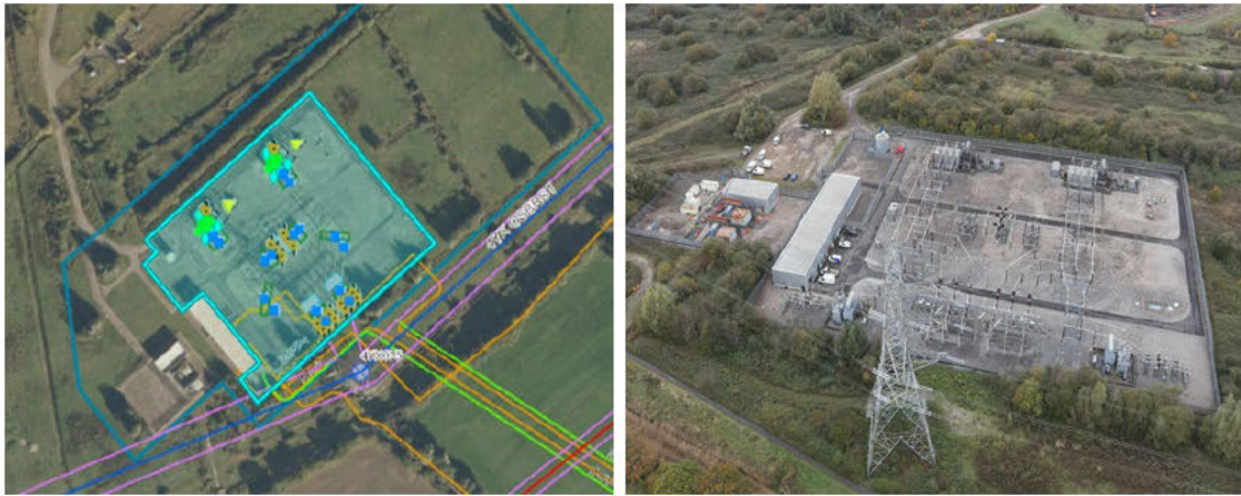
Figure 5: Aerial view of the Imperial Park substation
