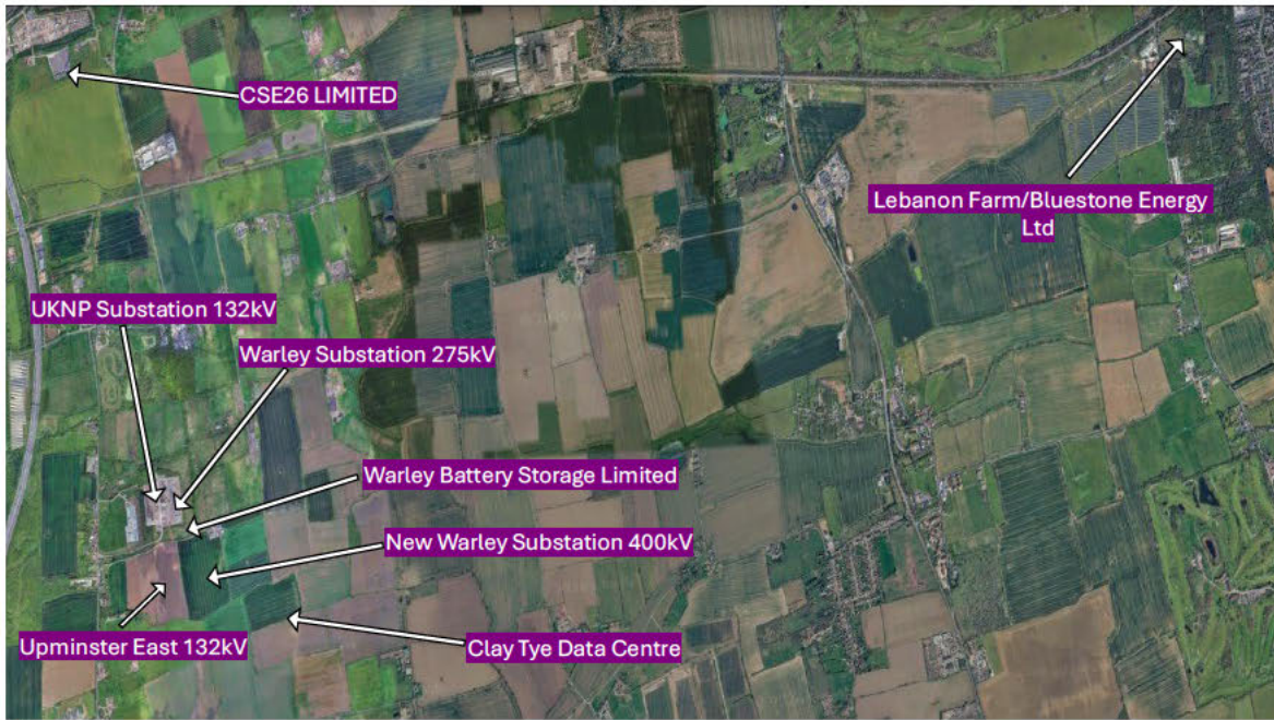
Figure 5: Existing Warley AIS 275kV Substation and adjacent 132kV [redacted] AIS substation
